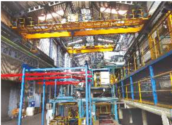
View of the new HPML plant at Koppal
